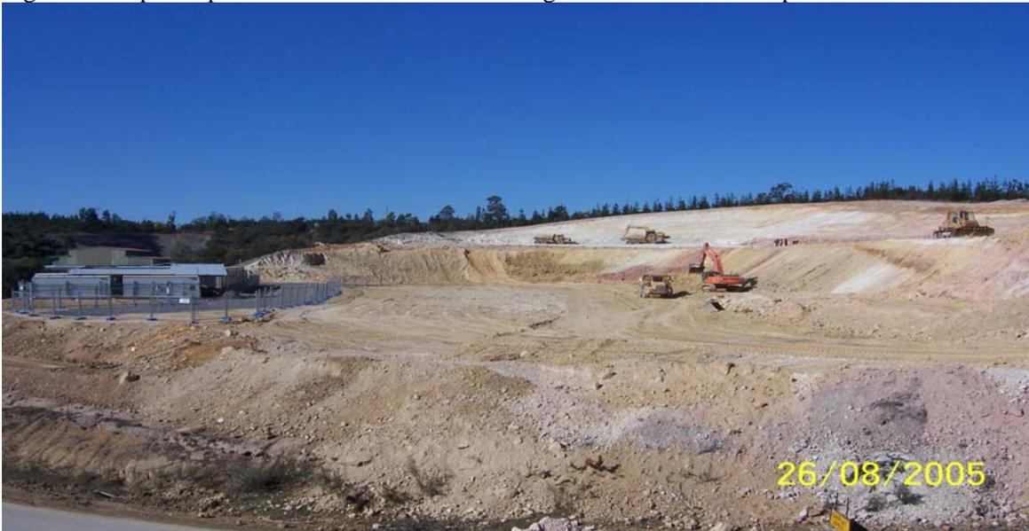
Figure 9: Benching at the BGF construction site
