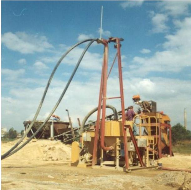
Figure 2: Installation of an IPJ with the tailings being pushed above the IPJ using the feed pressure.
