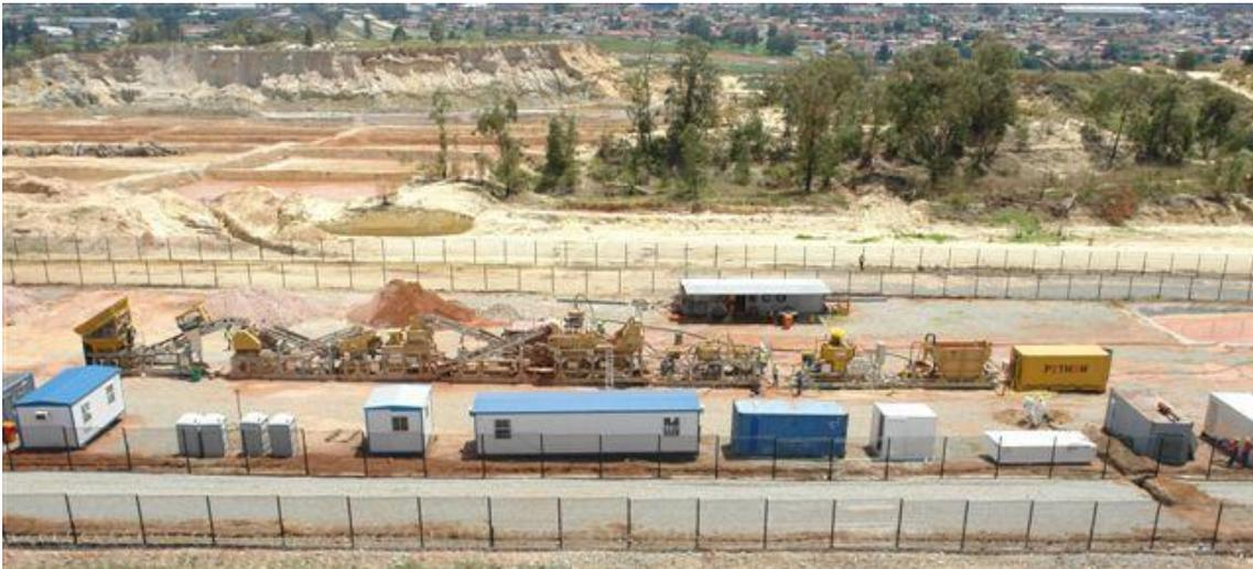
**Fig. 7.** Photograph of the Python plant operating at Central Rand Gold Limited in Johannesburg, South Africa. From left to right the modules are grizzly feed; primary crusher (jaw); primary screen and VSI; conveying; gravity separation (IPJ); flash flotation; water supply and MCC container.
